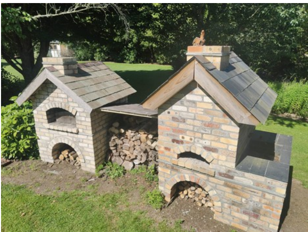
Matilda, wood-fired hot water and washing-up sink
